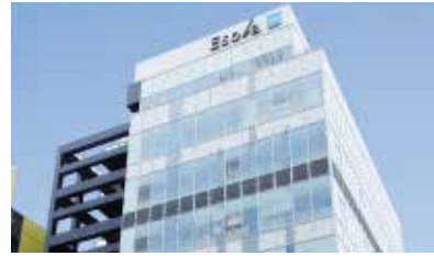
Commercial facilities in station building
