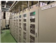
Stationary energy storage system
