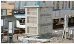
Station auxiliary power supply unit
