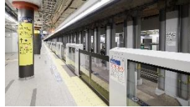
New station platform
