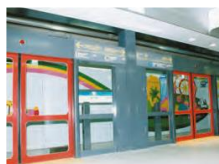
Platform screen doors
