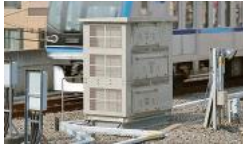
Station auxiliary power supply unit
